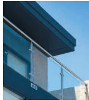
Coloured Cladding & Guttering
