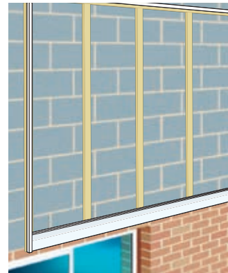
Fit first plank at base.
